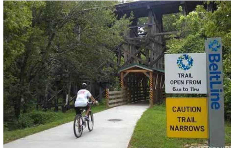
Canopy protective structure over trail when going under rail roads.
