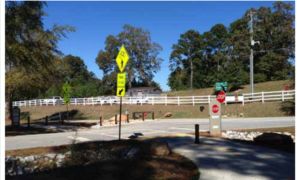
Typical trail intersection with signage, bollards, and pavement striping.
