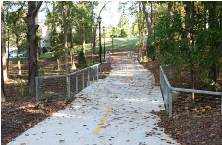
Custom steel bridge with handrail to span existing drainage swale.
