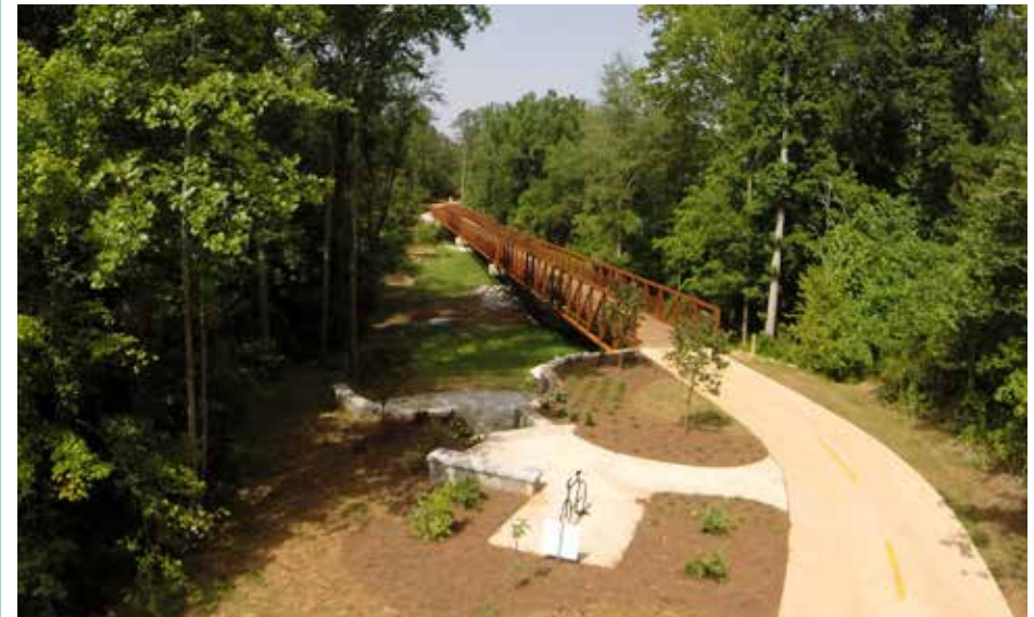
Prefabricated steel bridges allow trails to cross above existing roads and waterways.
