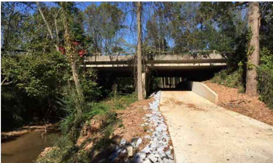
Multi-use trail going beneath an existing road bridge.
