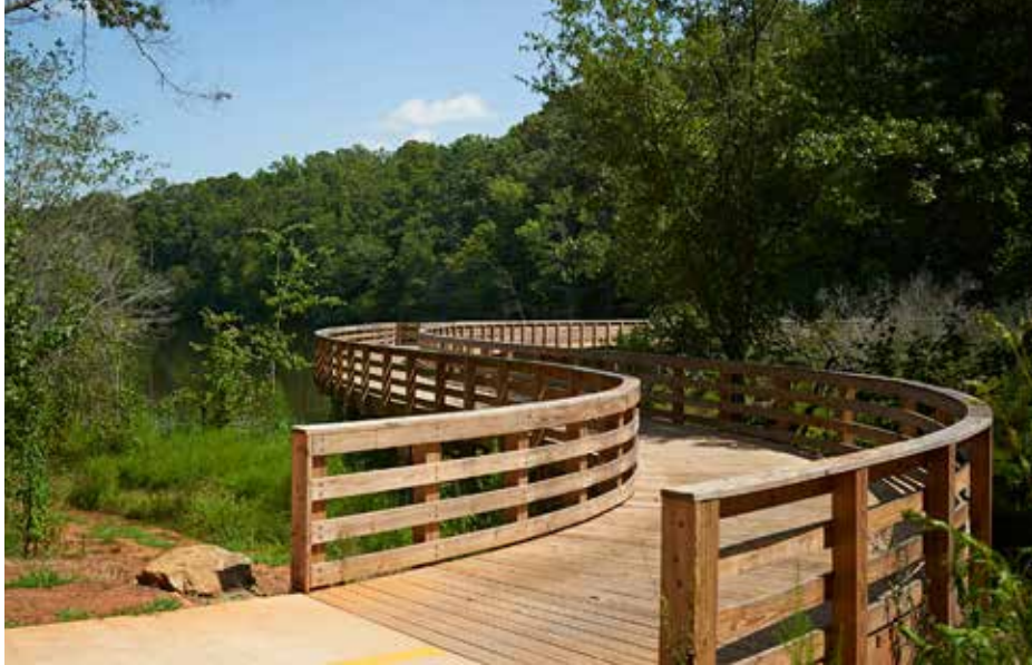
Wooden Boardwalk structure for crossing lakes and wetlands.
