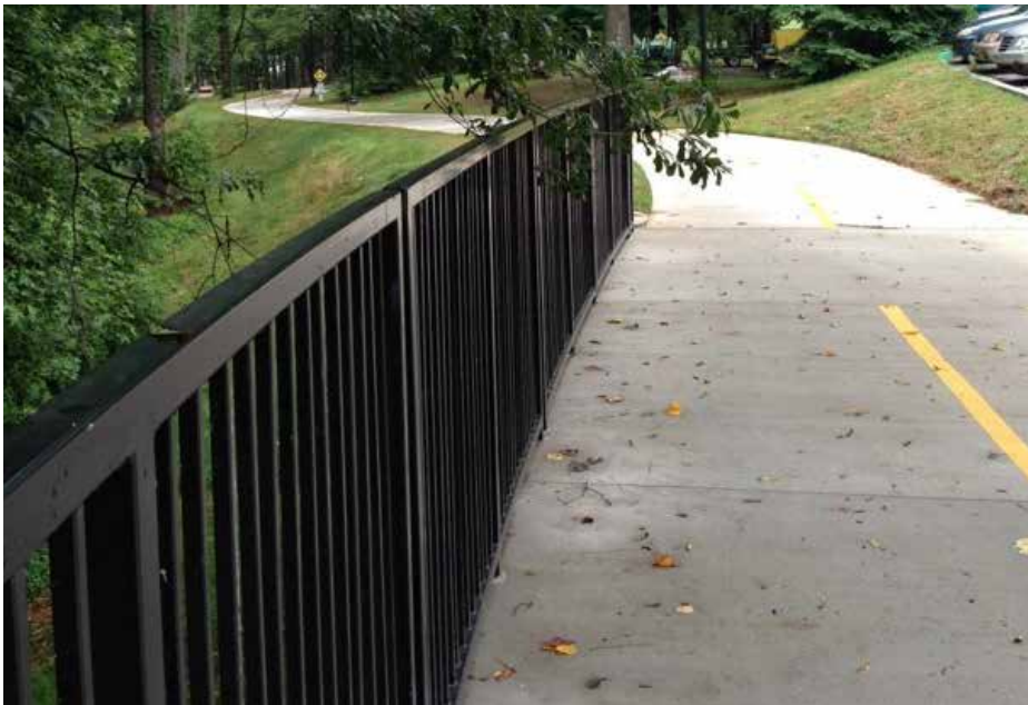
Black powder coated rail along a small bridged portion of the trail.
