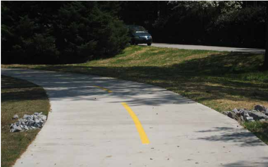
Structural slab constructed to allow drainage under the trail.
