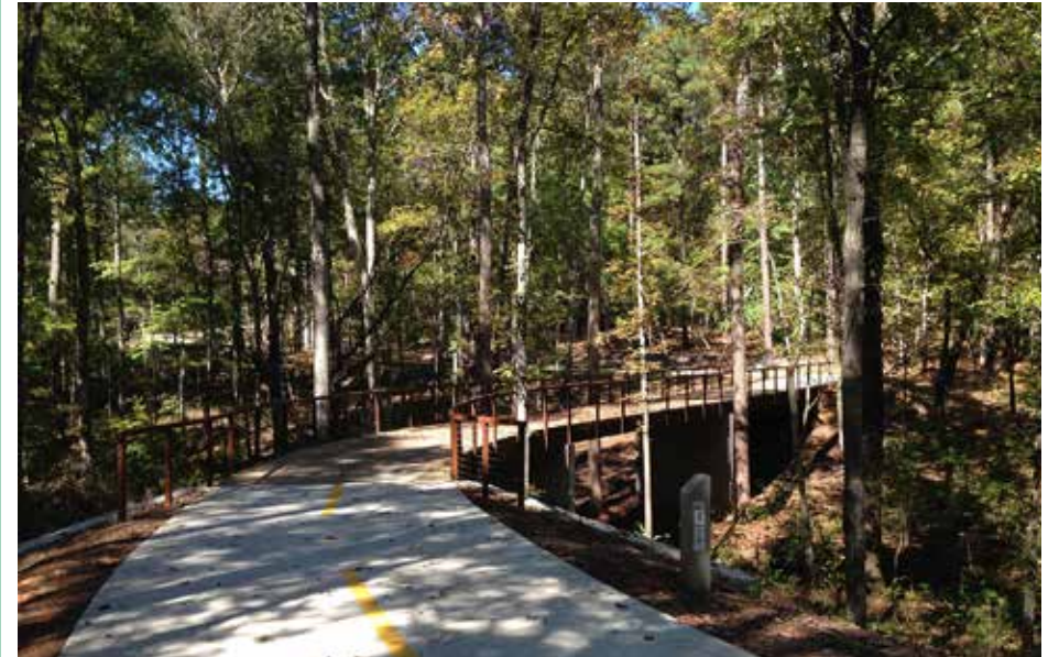
Custom steel bridge structures allow the trail to naturally blend into wooded areas.
