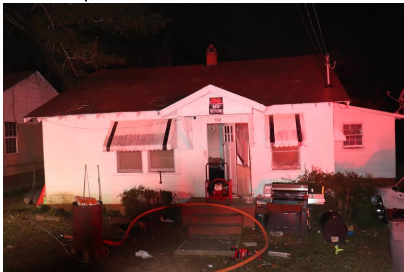
LFD responded to a fire on Milam Street
