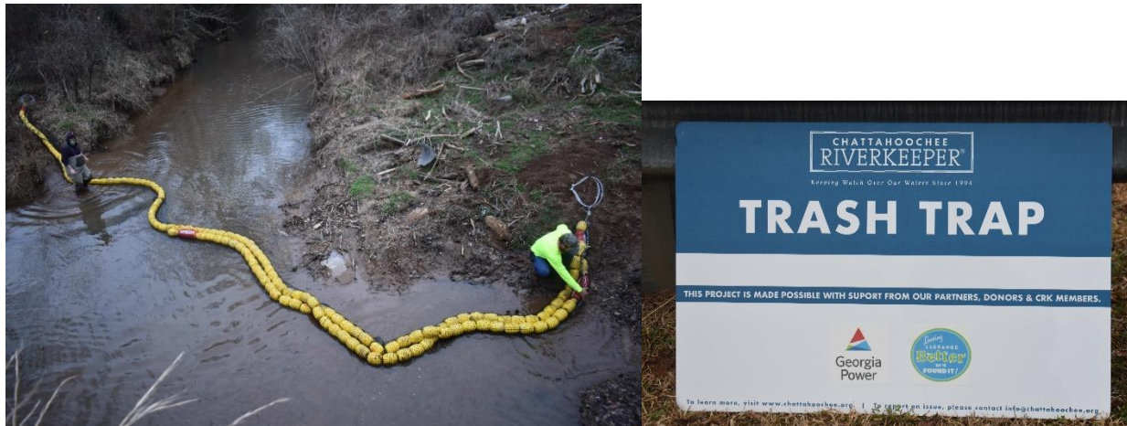
Trash Trap Installation at Dixie Creek
