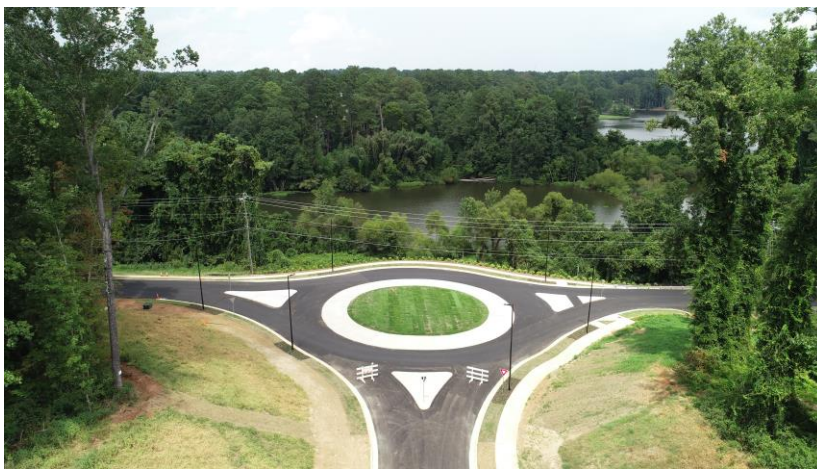
The new Country Club Road Roundabout/Hills & Dales Farm Road Intersection
