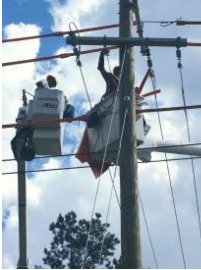
City of LaGrange Utility Workers in Blakely
