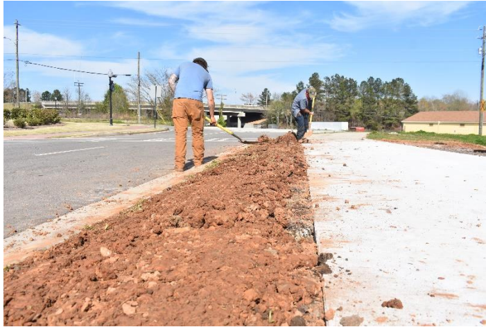
Crews continue to work on landscaping at the new skatepark
